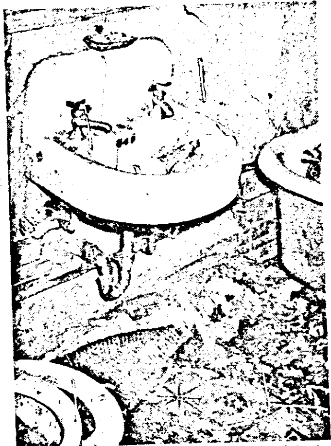
Workmen had begun repairing this bathroom before legal entanglements forced everything to a halt.
